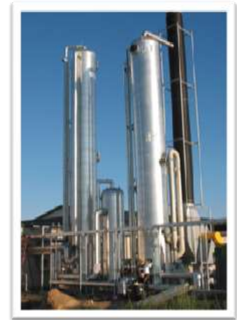
Fair Oaks, Indiana Totara+ System Installation
