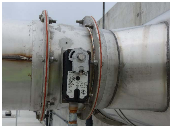
Figure 8: Damper & Actuator with score on end of shaft (closed position)
