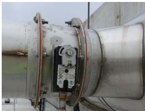
Figure 3: Aeration butterfly damper
