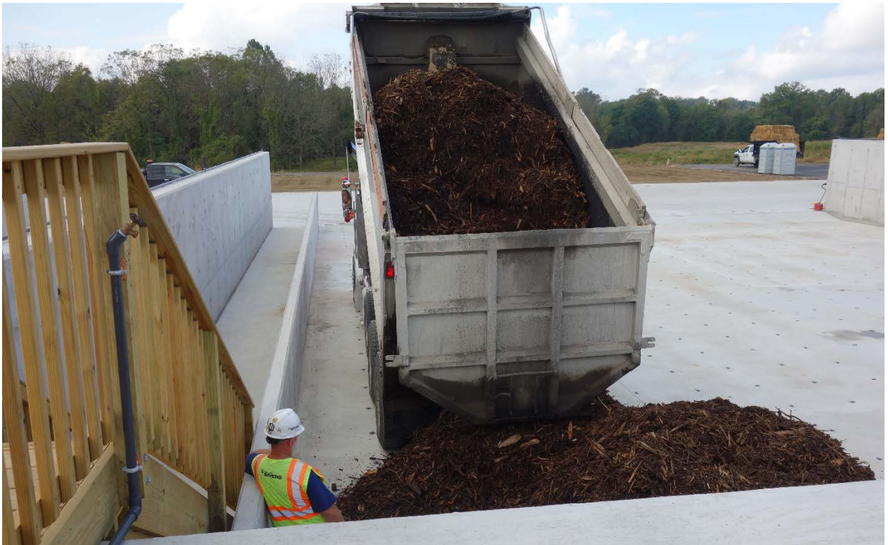
Figure 7: Biofilter media being installed
