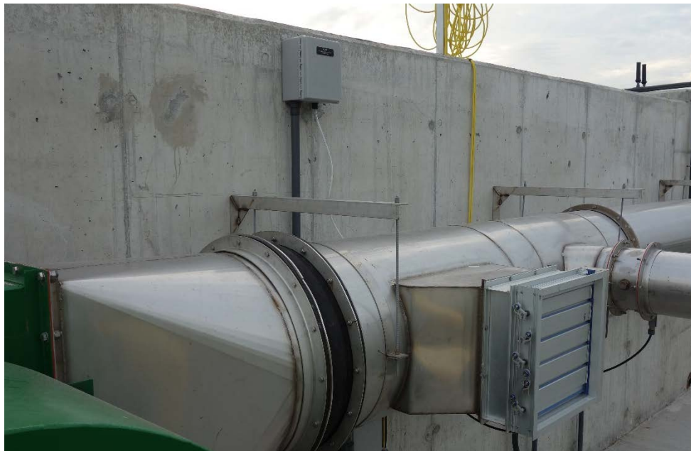
Figure 5: ECS Junction Box (mounted on wall) with pressure hose connected to aeration duct
