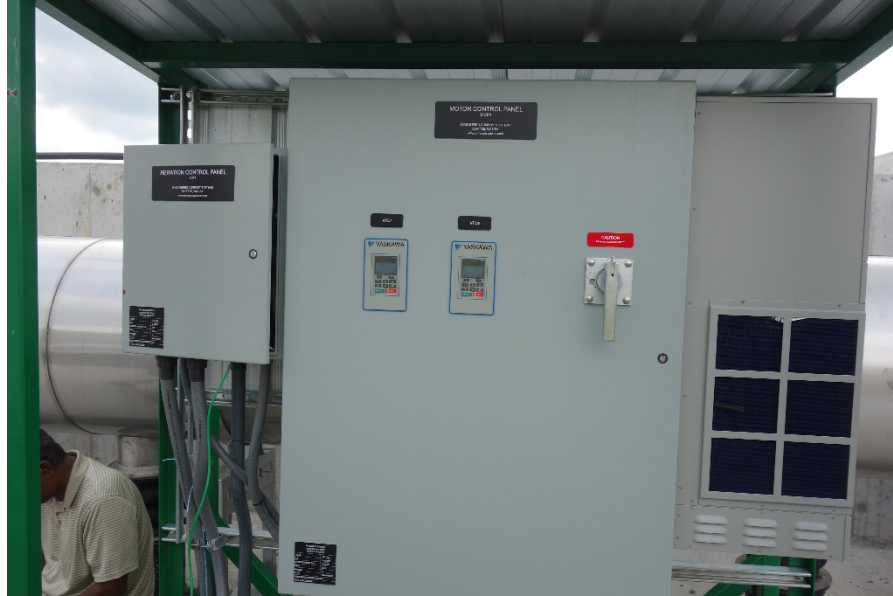
Figure 9: VFDs on Controls Skid
