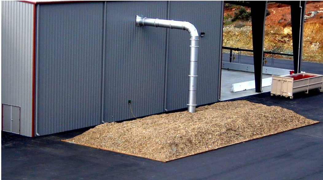
Biofilter with a Suspended Perforated Floor
