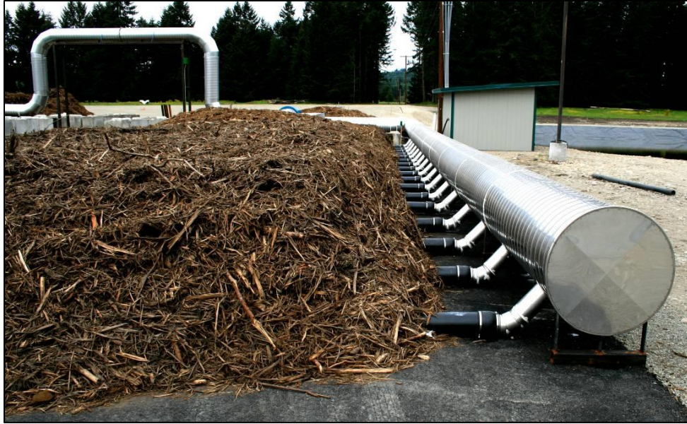
Figure 2: Biofilter with Above Grade Pipe and Coarse Media
