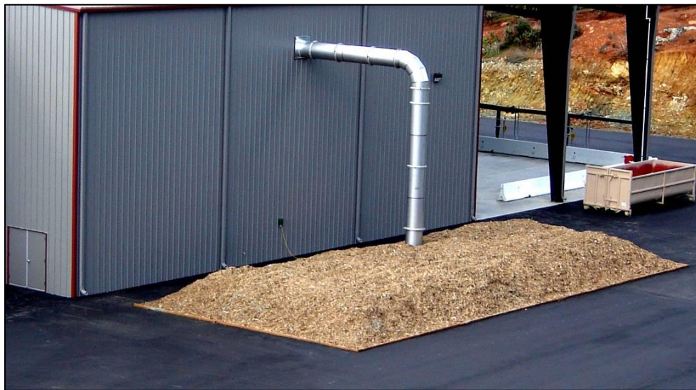
Figure 3: Biofilter with a Suspended Perforated Floor
