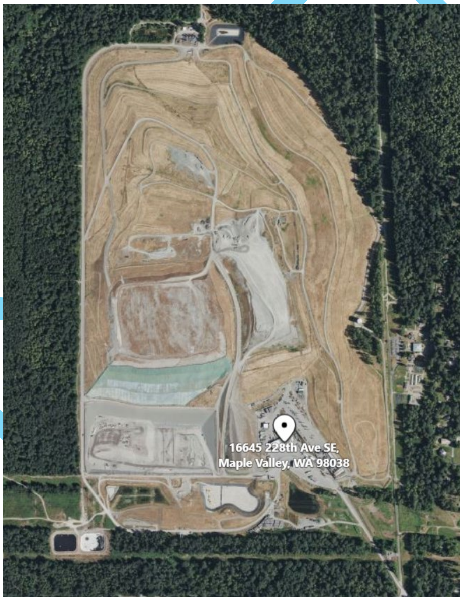
Aerial View of Cedar Hills Landfill – 2022
