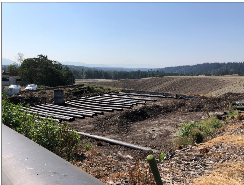
4. Lower Primary Biofilter and Ventilation System.
