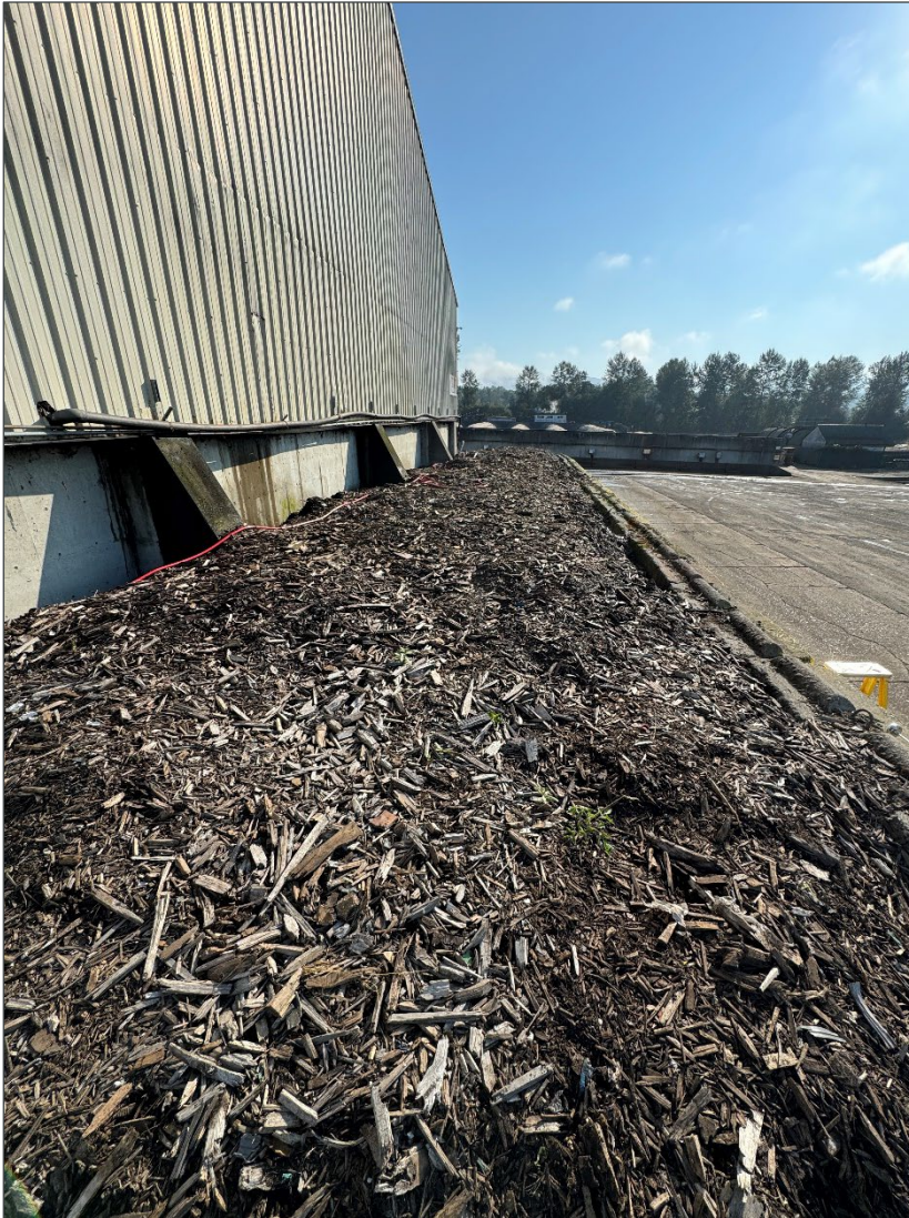
1. Tipping Building Biofilter.
