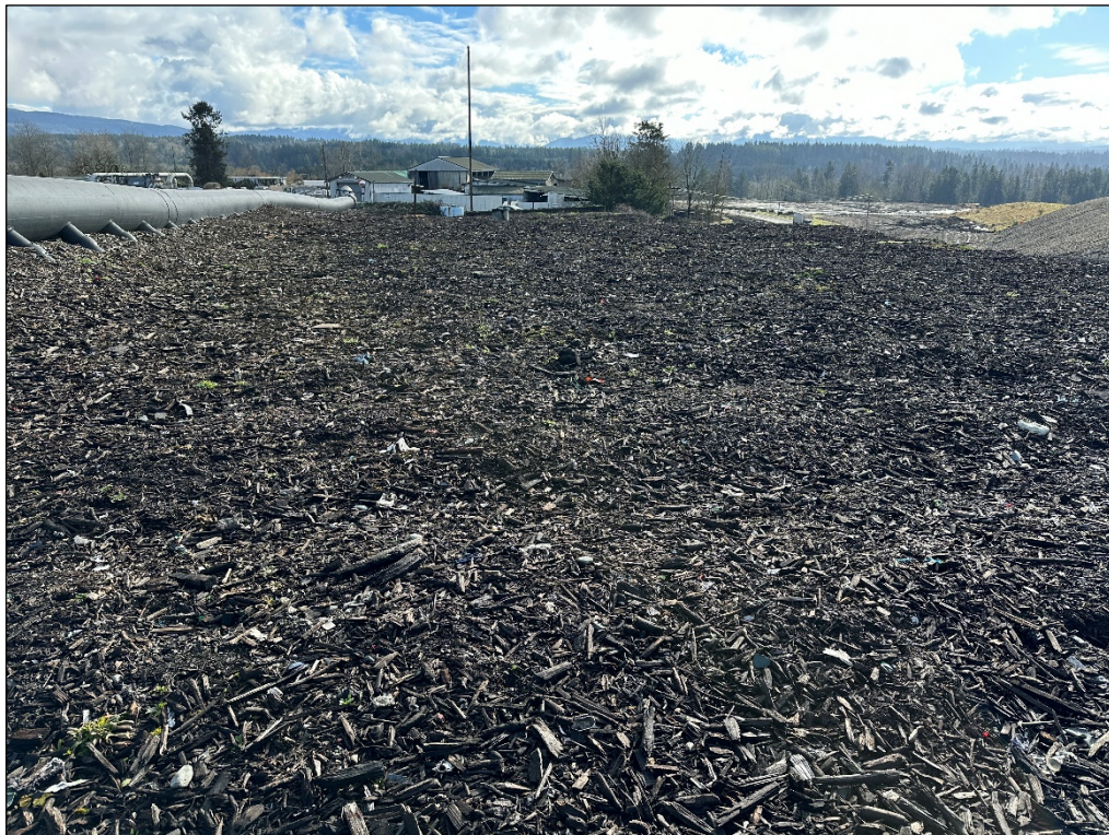
4. Lower Primary Biofilter and Ventilation System.
